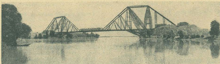
Most kolei North Western Railway w Indjach
